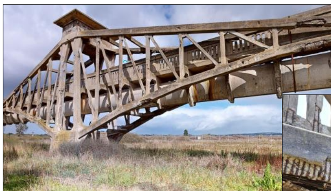
Top: Ovoid Sewer Aqueduct
