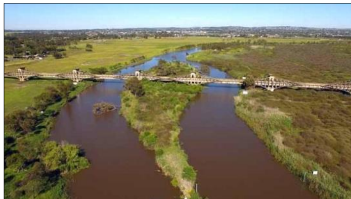
Aerial image of the Ovoid Sewer Aqueduct Photo: Courtesy of Barwon Water
